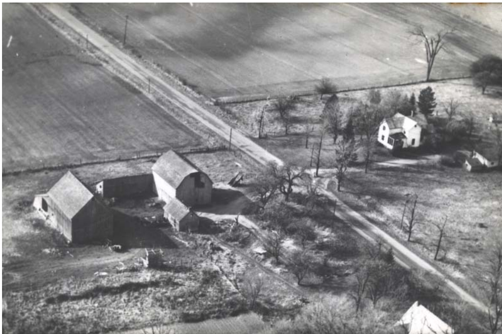
Arthur Andrews' dairy farm on North Road near Andrews Rd. The milk processing & bottling barn is the small barn in the center of the barnyard with the chimney on the near end, the drawing of which appears below.
